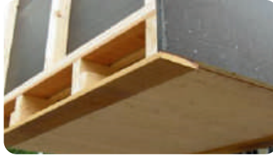
Difference in thickness between plywood and hardwood board.
