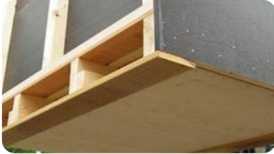
Pallet bottom closed by 9mm plywood.
